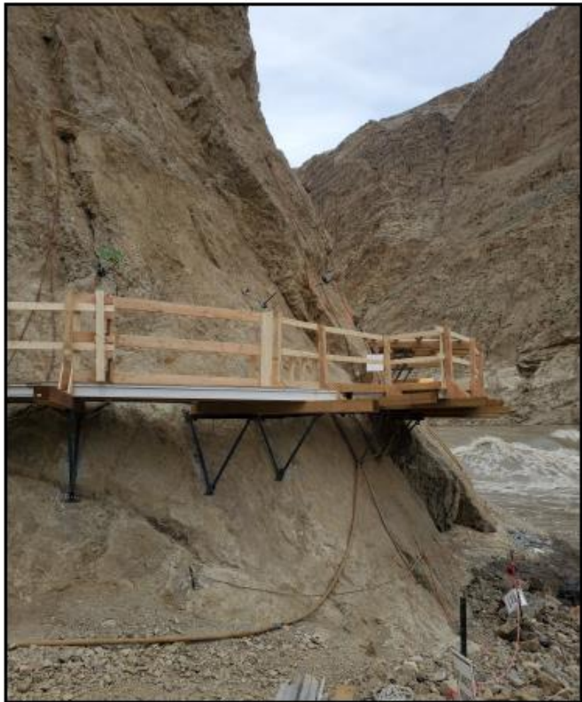
PICTURED: The working platform will help crew with the installation of the pneumatic fish pump system tubing.
