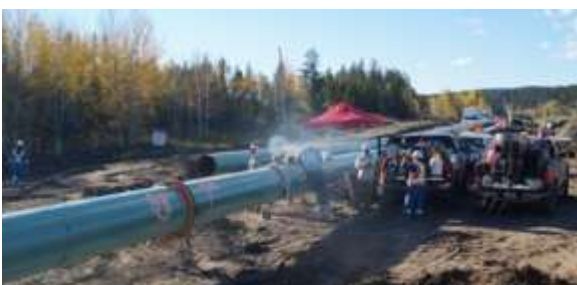
Figure 3: Welding new pipes
